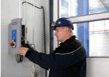
Our professional technicians service any brand of door.
